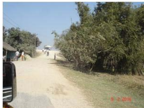
Village road Connectivity at EKE Ch. 76.80 km
