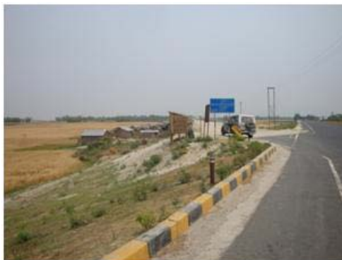
NH-57 Connectivity at EKE Ch. 31.90 km
